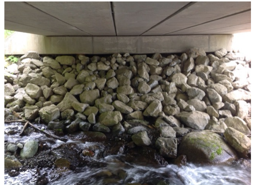
Left Bank Abutment when facing downstream
