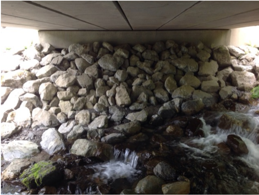
Right Bank Abutment when facing downstream
